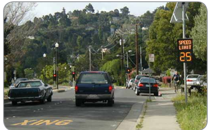
This solar-powered changeable message sign used in Mill Valley, CA is adjacent to a school and is only operational during the school commute periods. Image provided by David Parisi.
