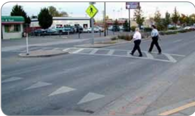
Painted triangles (shark's teeth) are used as the yield line at unsignalized locations.
