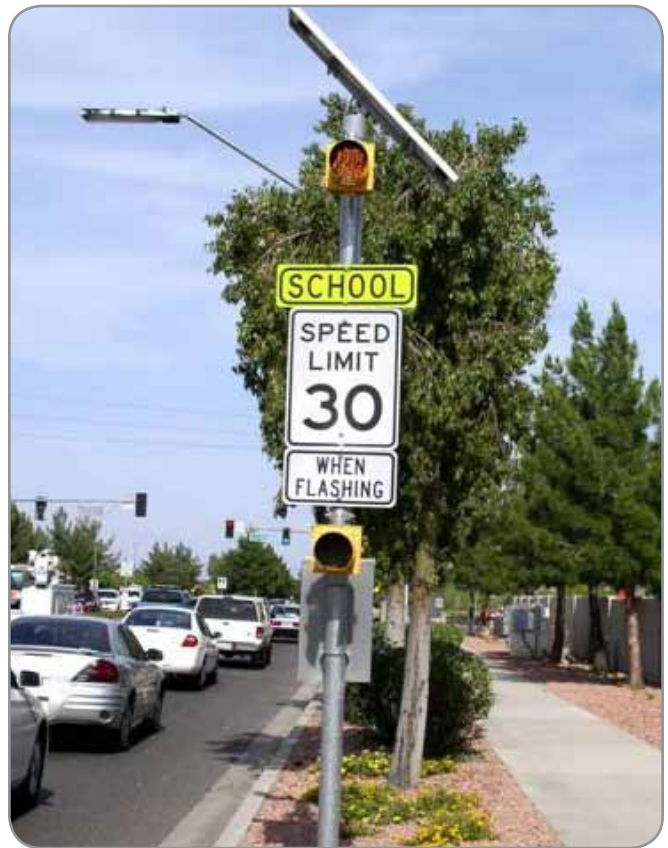
School flasher speed limit sign at Arrowhead Elementary School in Glendale, AZ. Image provided by Mike Cynecki.
