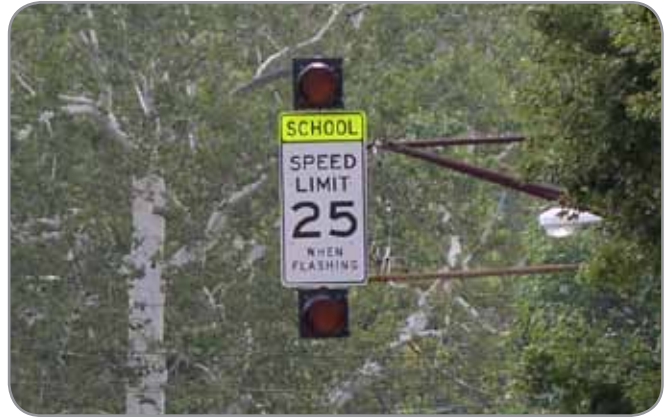
Overhead school flasher speed limit sign at Second Street School in Frankfort, KY. Image provided by Mike Cynecki.
