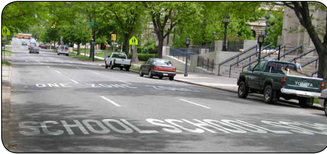
Pavement markings at Morey Middle School in Denver, CO. Image provided by Mike Cynecki.
