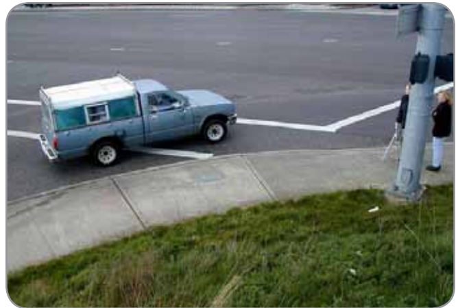
A large turn radius allows drivers to make higher speed turns and increases the crossing distance.
