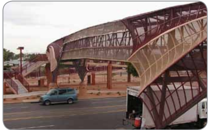
Pedestrian bridge at Isaac Middle School in Phoenix, AZ. Image provided by Mike Cynecki.
